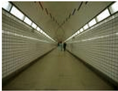
Figure 5: Tunnel lighting (outside the product boundary)
