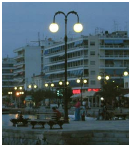
Figure 41: Example of a luminaire that was excluded from this improvement option, reason: too much upward light, little directed to walking lane and light loss in the opal diffuser.
